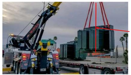
For unloading, lifting hooks are provided near the top of the transformer tank. When slings are being used to lift the MVT's, the sling pull angles should **not be over 30°** from the vertical axis refer to left side picture (red reference line; vertical axis).
