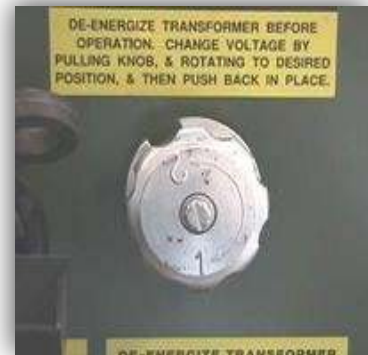
Figure 9 – Linear multi-voltage switch
