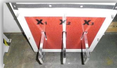
Figure 4 - Typical Busbar
