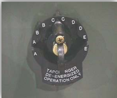
Figure 5 – Rotary Tap Changer
