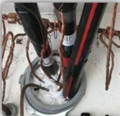
Figure 15 - Sealed Cables
