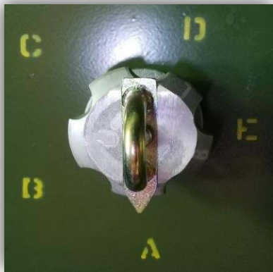
Figure 7 – Linear TC with Hotstick Handle
