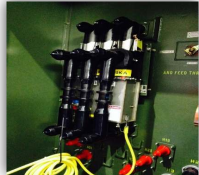
Figure 12 - Molded Vacuum Interrupter
